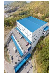
Icheon Maegok DC Logistics Center
