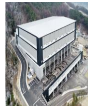
Icheon Hoieok-ri Logistics Center
