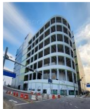
Greenwave Siheung Logistics Center
