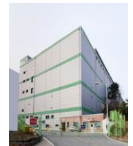
Myungse Logistics Warehouse
