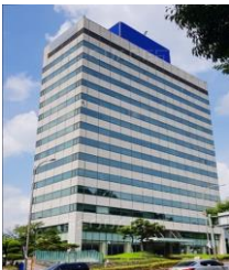
GS Construction Seocho Tower
