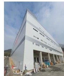
Wide Creek Bangchori Logistics Center
