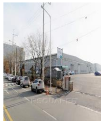
Wonjeong-ri General Logistics Center
