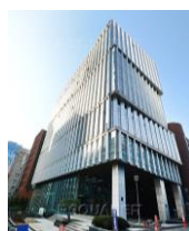
Yeoju Bonduri Logistics Facility
